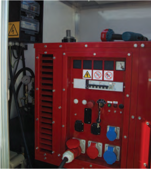
Electrical generator inside B-10
